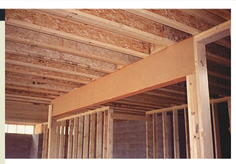
lumber. Careful consideration needs to be taken where and how it is cut. "Holes less than 1.5 inches diameter are generally okay as long as they're not on, or into the flange. Drilling through the web material is normally an acceptable practice," says, O'Day.
